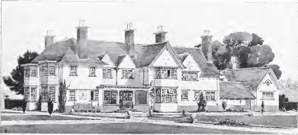
House on Beacon Hill, Penn, Bucks , F. A. WHITWELL, Architect. (For Plan, see p. 127.) Contractors: Webster and Cannon, Aylesbury.
